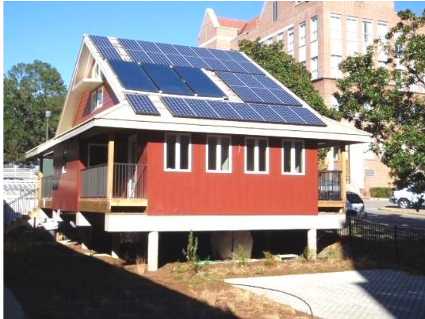
Figure 5: South facing roof of OGZEB
