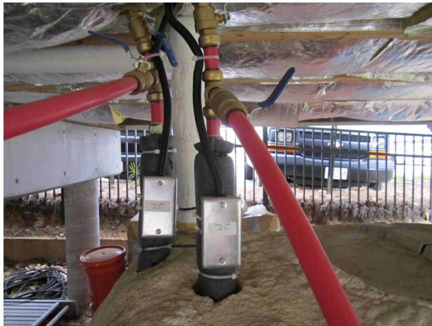
Figure 8: Wrap around pipe temperature sensors
