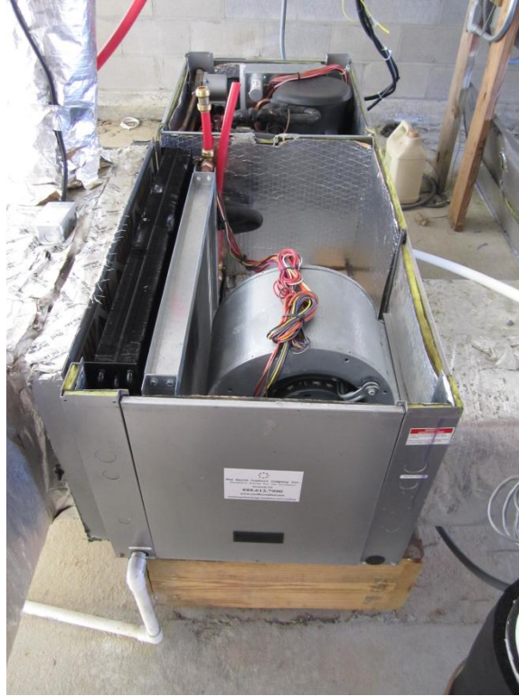
Figure 14: Side view of heat exchanger
