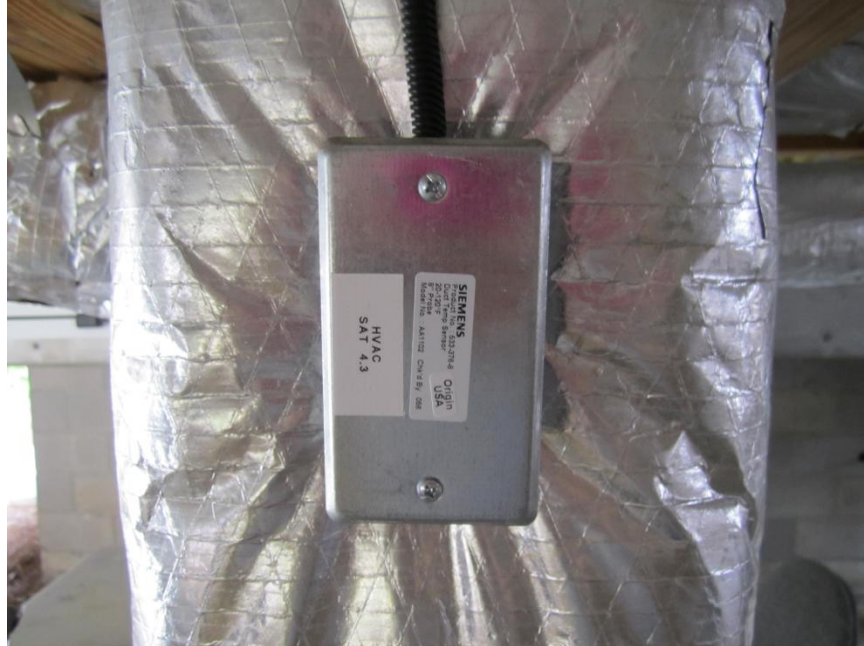
Figure 9: Duct temperature sensors
