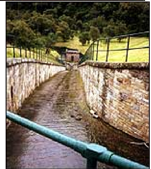
spillway chute from side channel to river
