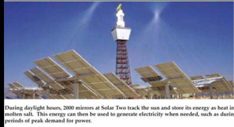
**Power Tower** systems use a circular field array of heliostats (large individually-tracking mirrors) to focus sunlight onto a central receiver mounted on top of a tower (Figure 2). The first power tower, Solar One, which was built in Southern California and operated in the mid-1980's, used a water/steam system to generate 10 MW of power. In 1992, a consortium of U.S. utilities banded together to retrofit Solar One to demonstrate a molten-salt receiver and thermal storage system.
