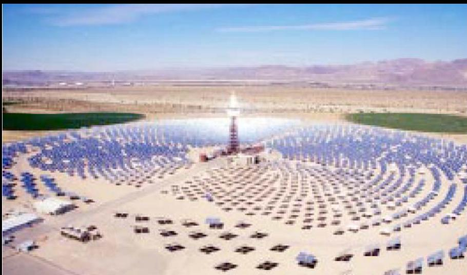
**Power Output:** Solar Two produced 1633 MWh over a 30-day period, exceeding its one-month performance measure of 1500 MWh of power production; the plant also produced a record turbine power output of 11.6 megawatts.
