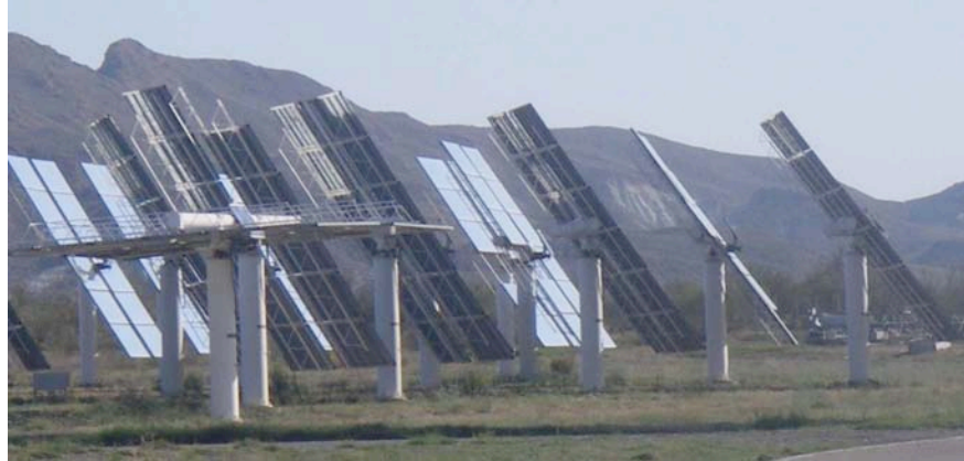
Figure 24. Typical advanced heliostat field. (source: Plataforma Solar de Almeria - PSA, Spain)
