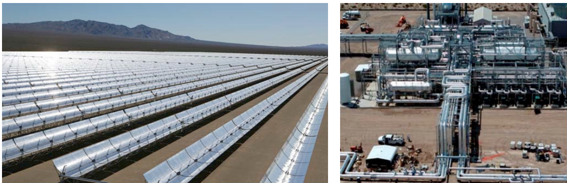
Figure 12. Left: Parabolic trough field; Right: Power block at Nevada Solar One Power Plant. (Source: www.acciona-na.com )
