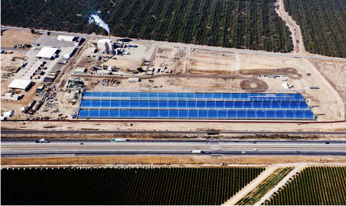
Figure 19. The Ausra 5 MW Kimberlina solar thermal demonstration plant. (source: http://www.ausra.com )
