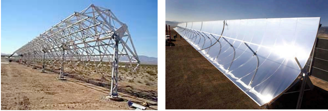
Figure 8. Left: Parabolic trough space frame structure (Source: NREL); Right: Lightweight trough with reflective thin film mirror (Farr &Gee, 2009).
