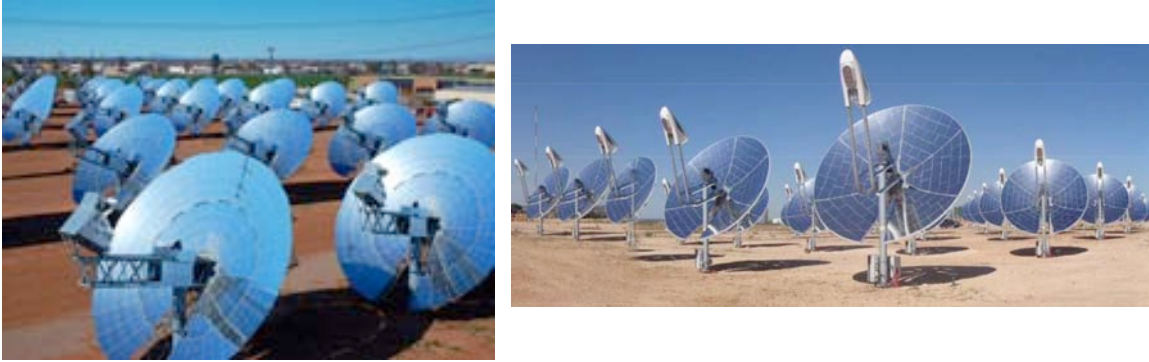
Figure 22. Left: 1.5 MW Maricopa Solar installation (source: http://www.srpnet.com/maricopasolar ); Right: 1 MW solar installation in Villarrobledo, Spain (source: http://www.infiniacorp.com ).
