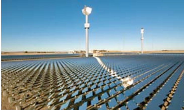
Figure 27. 5 MW twin central receiver tower facility with 1 m 2 heliostats in California. (source: eSolar)
